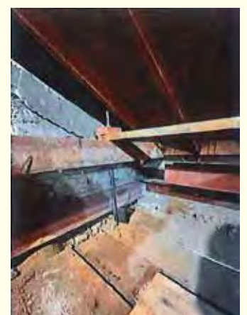
Steel rod and beam installation.
