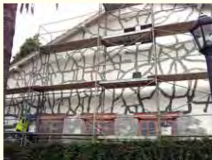
South wall repairs.
