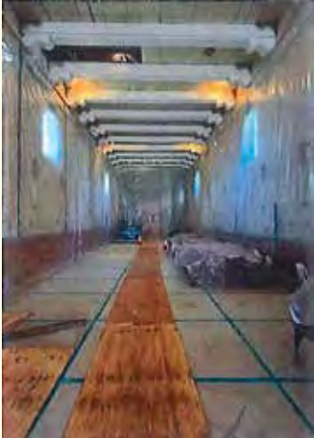
Interior of the church is protected and floor is covered.
