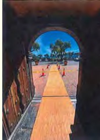
Interior tiles and exterior pavers are protected.
