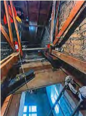
Worker in attic.
