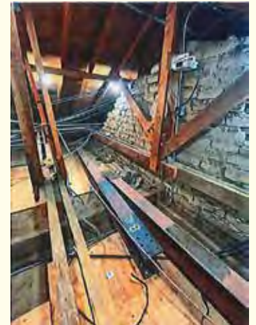
Beams ready for placement.
