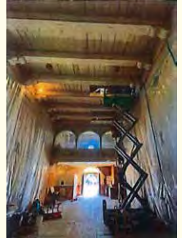
Ceiling access is by lift.
