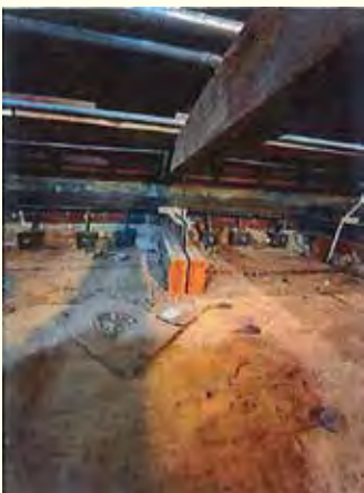
Installed L brackets.
