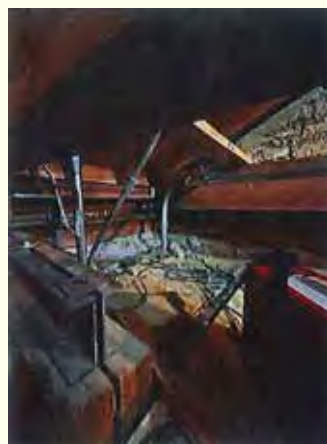
Beam ready to be installed.
