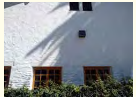
Completed south wall.
